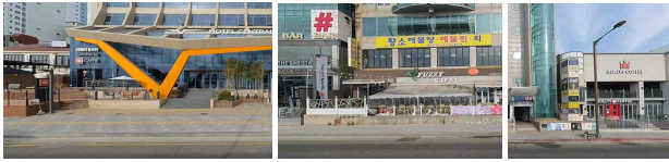
a) raised deck in front of hotels b) decks of commercial buildings c) flood barriers
